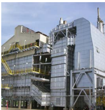
REKULUVO with reactor and duct in a methanol plant
